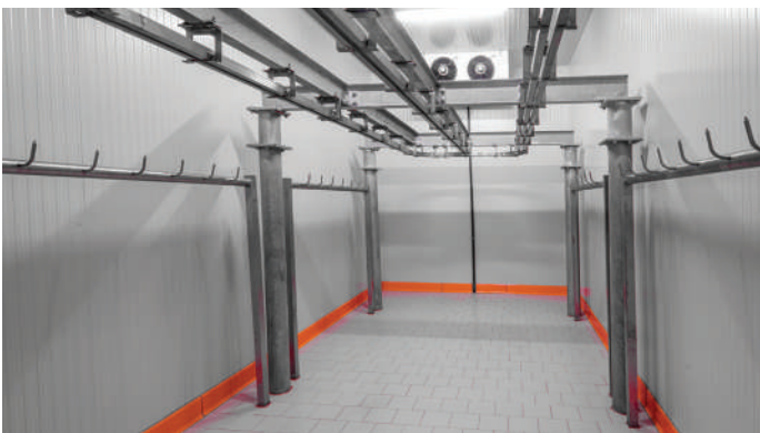
Cold Room and Storage
