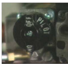
Turn gas valve to Pilot.
