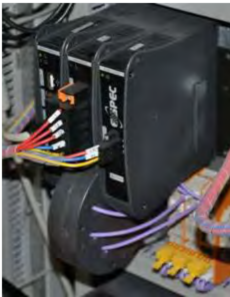
G4K Successful Current Wiring
