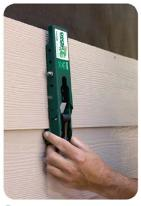
of your siding's overall length from either end, place the Gecko's blade under bottom edge of siding and slide upward.
