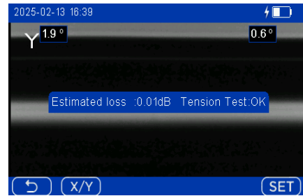
Completed splice with estimated loss
