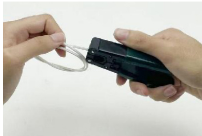
Stripping protective layer from drop cable
