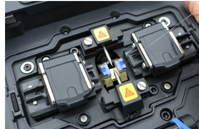
Remove debris from V-grooves
