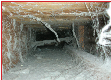
Inspection of hard-to-reach and hard-to-see areas
