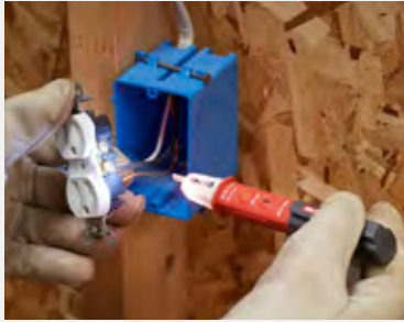
Test wires for AC voltage
