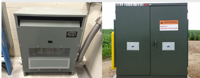
Custom replacement dry transformer panel-front with a built in maintenance inspection window
