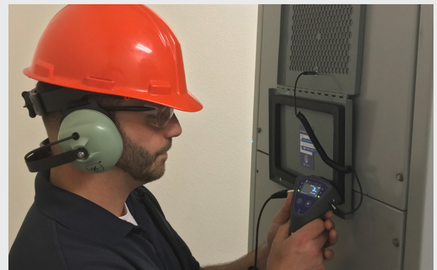
With a maintenance inspection window for visual, infrared, ultraviolet, and ultrasound inspections installed on medium voltage switchgear, no special PPE is required to use the EMSD
