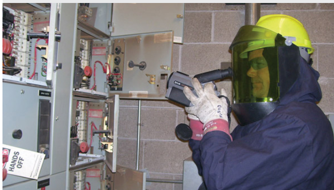
Infrared scanning is applicable on all electrical assets including motor control centers, but typically requires extensive PPE if done “open panel”
