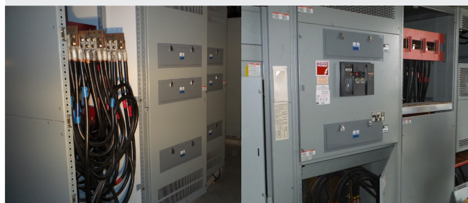
Incoming line connection and main breaker cabinets were also fitted with 24-inch windows
