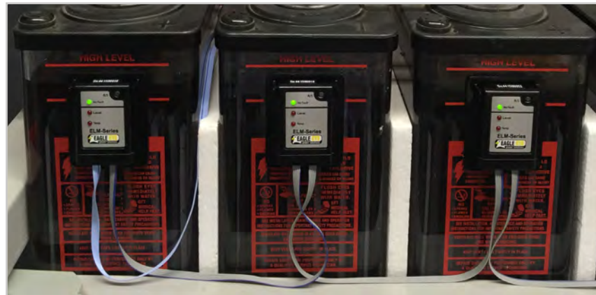
Sensors Installed to Level Line on Flooded Cells
