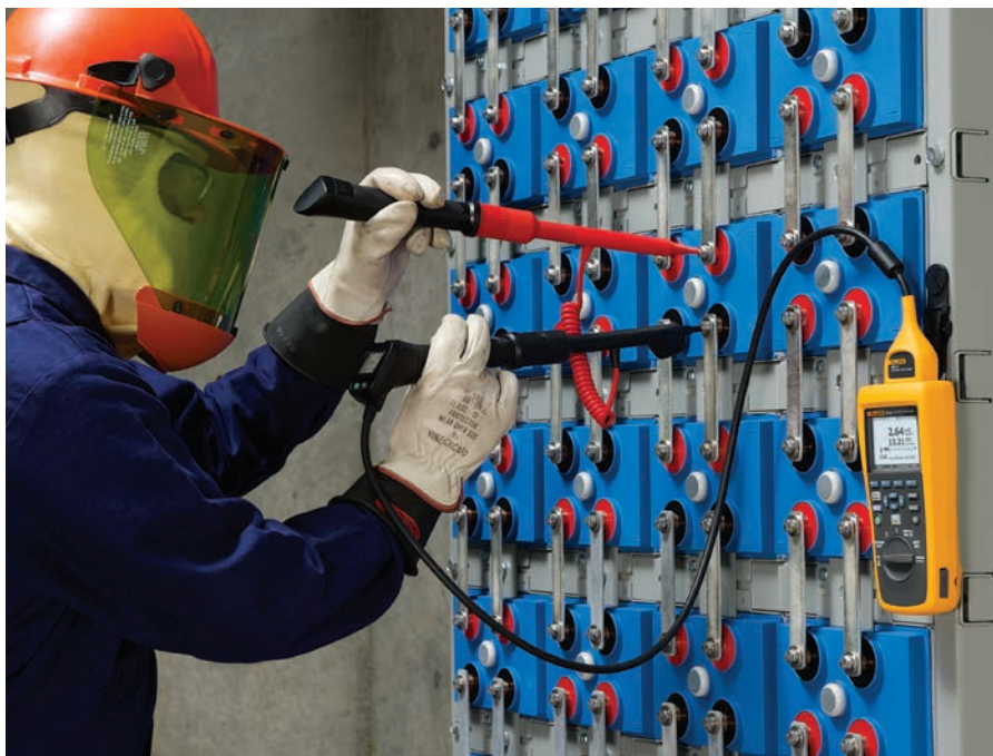
Measuring ohmic values in sequence mode
