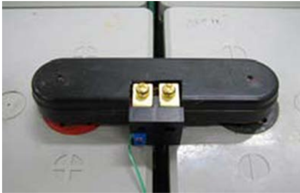
C-Type Clamps Installed to Busbars
