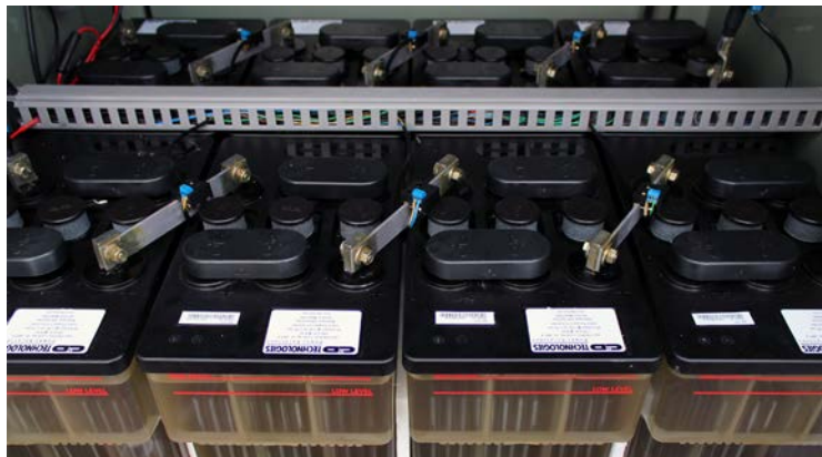
Duct Installation on (8) 6V Jars
