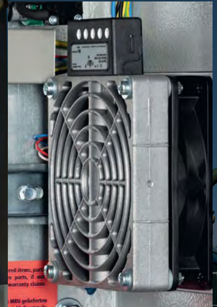
Cabinet heating temperature regulated, for use in environment from -5^{\circ}\text{C}
