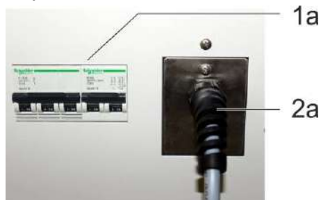
Safety cutouts and mains cable at A80t
