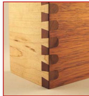
Cuts Through Joints
