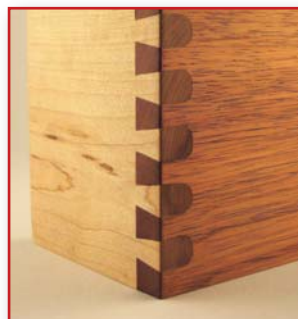
Cuts Through Joints
