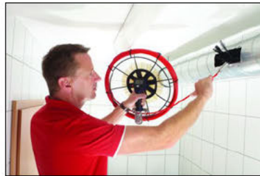
Fig. 21: Cleaning a ventilation duct
