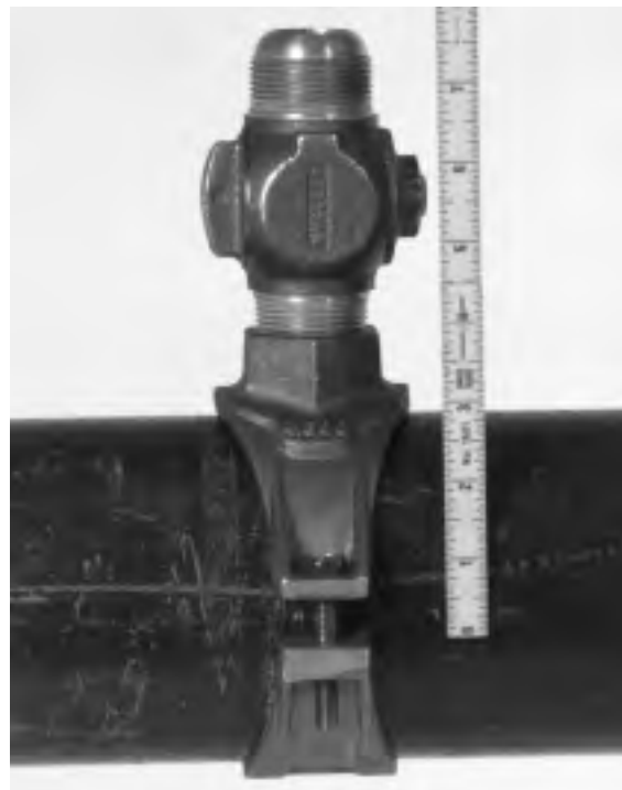
Figure 9 – Measuring valve standoff distance
