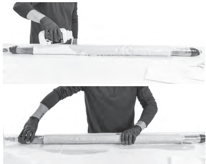
Figure 33 – Wetting Out The Patch On The Packer
