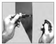
2 Place 1/2" conduit die on 3/8" draw stud. Insert draw stud through pilot hole.
