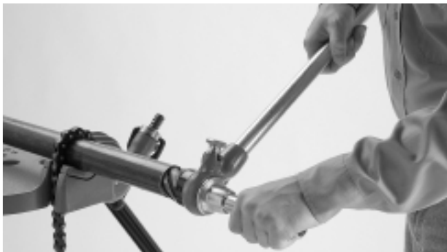
Figure 2 – Reaming End of Pipe
