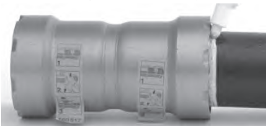
Figure 7 – Marking the Pipe After Fully Inserting Pipe
