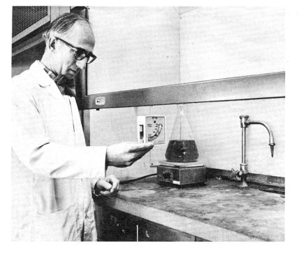
Use a Vaneometer to measure velocity of air flow into laboratory fume hoods and...
