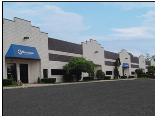
European Sales Office and Warehouse
