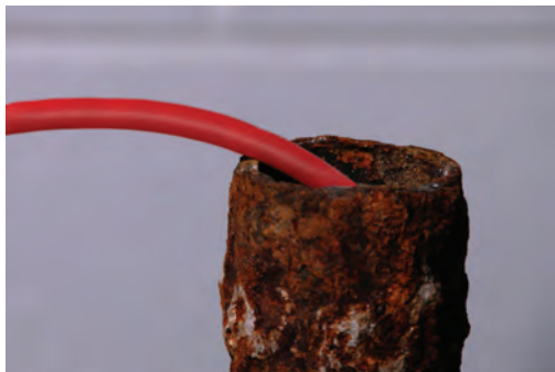
Figure 16 – Avoid Pulling at Sharp Angles
