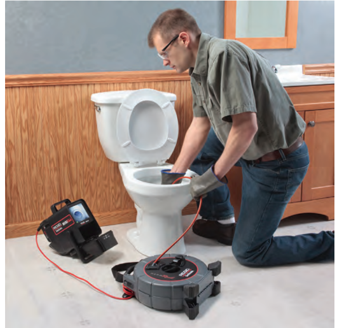
Figure 14 – Performing an Inspection
