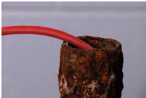
Figure 16 – Avoid Pulling at Sharp Angles
