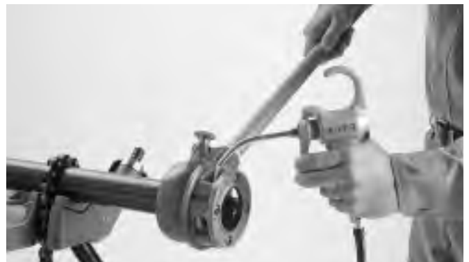
Figure 4 – Applying Thread Cutter Oil
