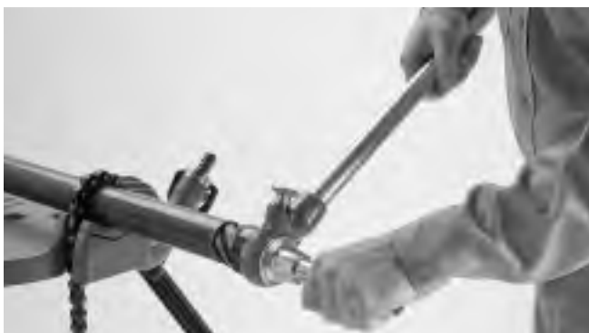
Figure 2 – Reaming End of Pipe
