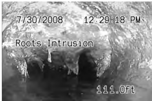
Figure 25 – Display Screen with Slide Text, Time and Distance Shown (Distance measured from system zero-point)
