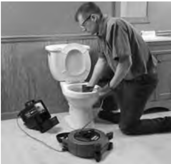
Figure 15 – Doing An Inspection
