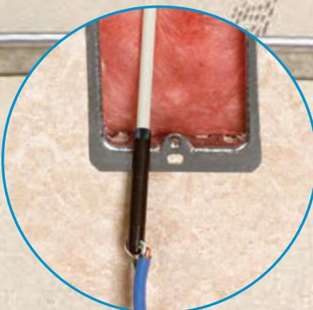
**Tuff-Rod™** is an excellent choice for pulling wire where insulation is already installed.
