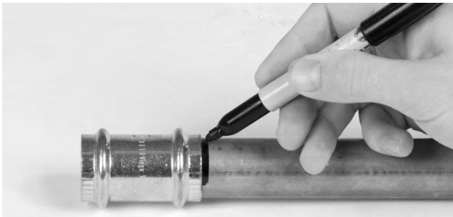
Figure 8 – Marking the Tubing After Fully Inserting Tube
