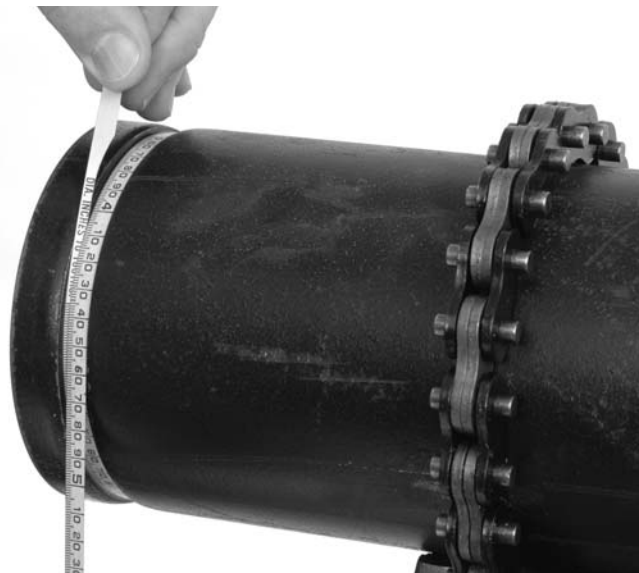
Figure 11 – Checking Groove Diameter With A Diameter Tape
