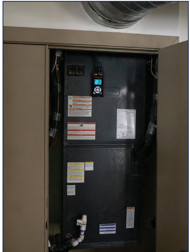
In this study, the load analysis was conducted using the AEMC® Instruments PEL 52. To secure the device in place during the week-long testing period, four powerful magnets on the casing allow it to be easily attached to the flat metallic surface of the HVAC system.
