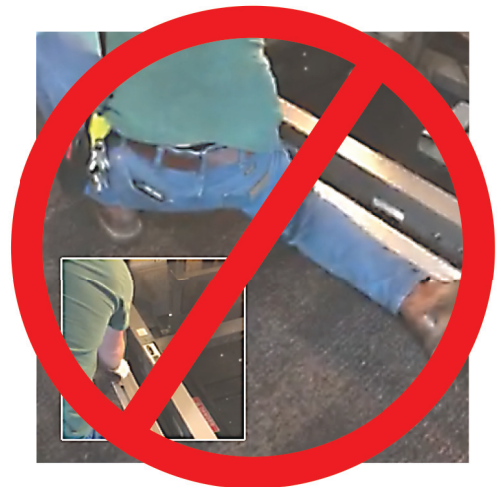
No need to crouch to set wedges while holding doors with your feet.
