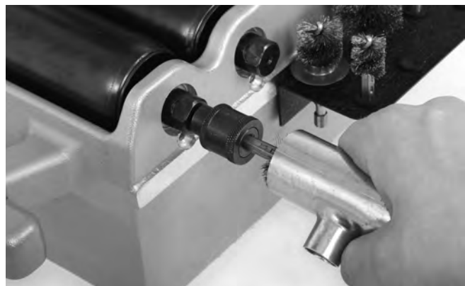
Figure 14 – Cleaning Inside of Fittings
